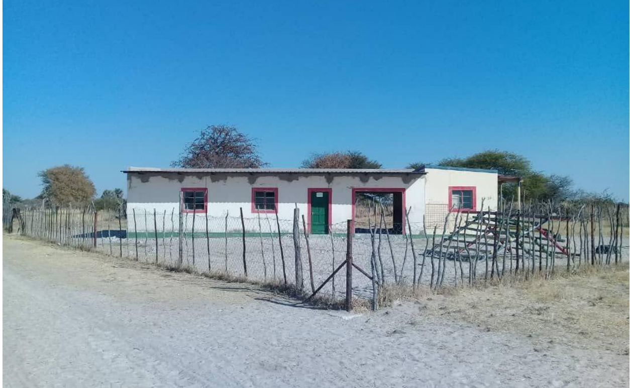
The kindergarten building after the finished repairs
